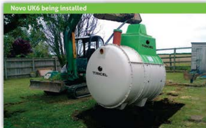
Novo UK6 Wastewater treatment plant installed
