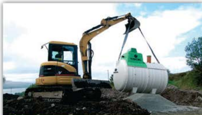
Novo UK6 being installed
